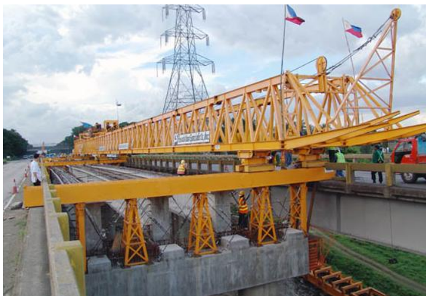
Example of Portal Beam and I-Girder Installation
