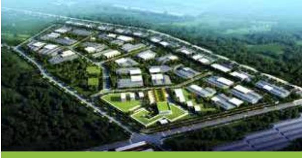
National Special Economic Zone (under construction)
