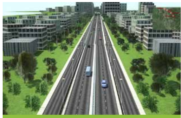
Dhaka Bypass Expressway (under construction)
