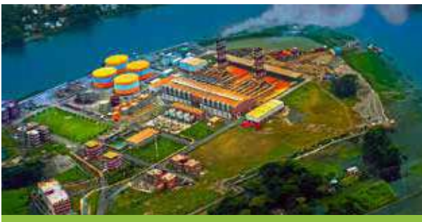
Desh Energy Chandpur Power Company Limited
